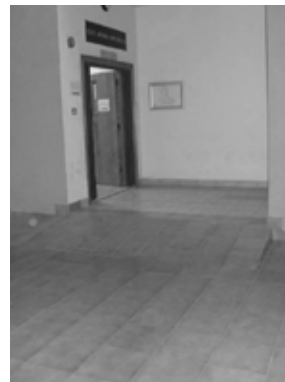
Figure 6: Gentle ramps at the refectory and bookstore but no rails
