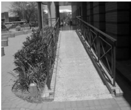
Figure 2: Good gradient shaded ramps with handrails and non-slippery flooring – Administration building
