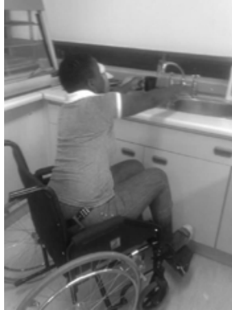
Figure 12: High counters and no knee space at the food laboratories
