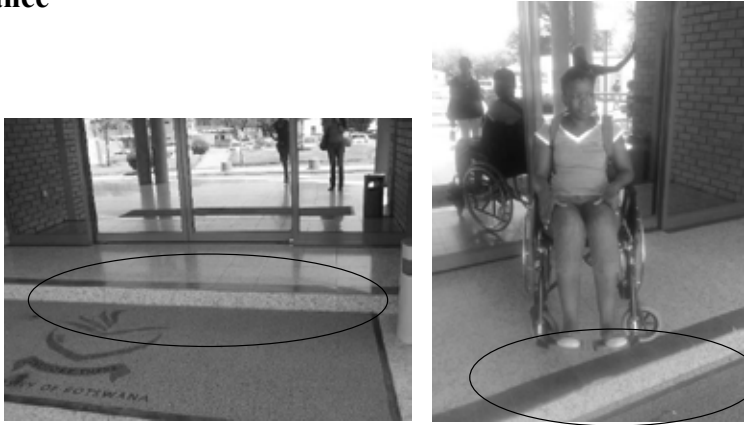
Figure 3: No ramp or threshold at the Administration building entrance
