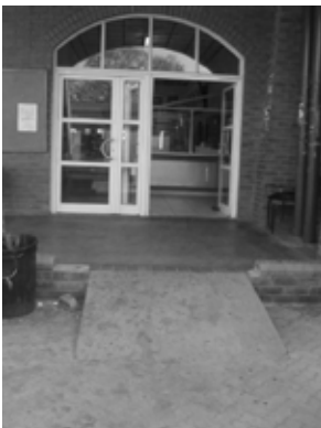
Figure 6: Gentle ramps at the refectory and bookstore but no rails
