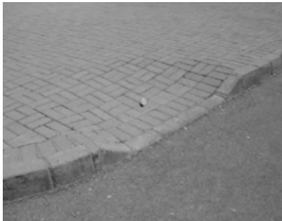
Figure 8: A well maintained and not so well maintained dropped kerb
