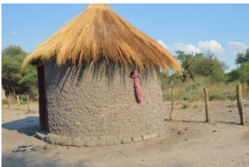
Figure 4-3: Hut built out of termite mound clay and thatched with Cymbopogon caesius . Habu village November 2016
