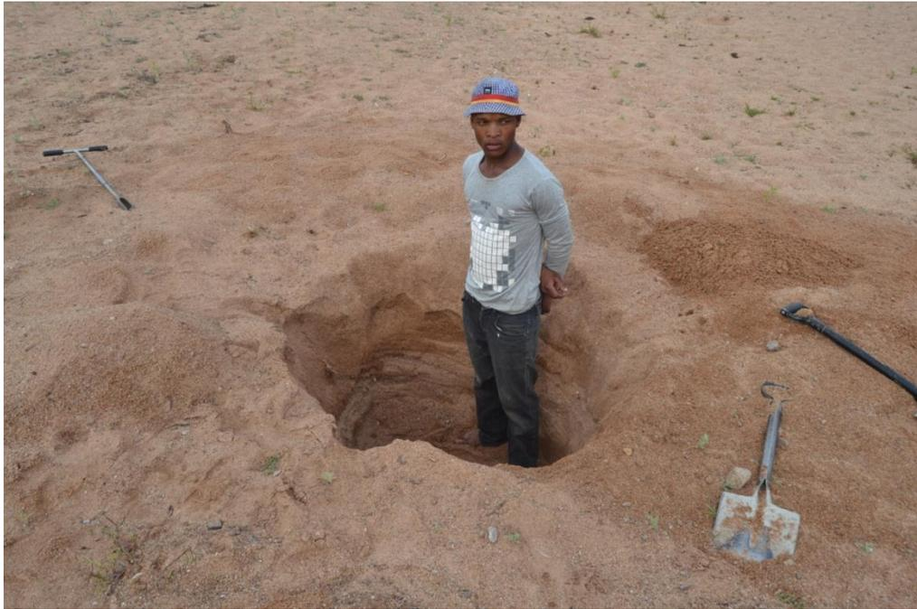
Figure 16: A 1m hole dug in the riverbed before auger installation
