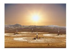
Figure 6: Tracking plane mirrors mounted in a large field reflect solar radiation on to a central receiver atop a tower.
